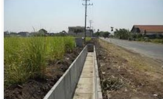
Benahi Infrastruktur Drainase 2019 ... kalsel.antaranews.com
