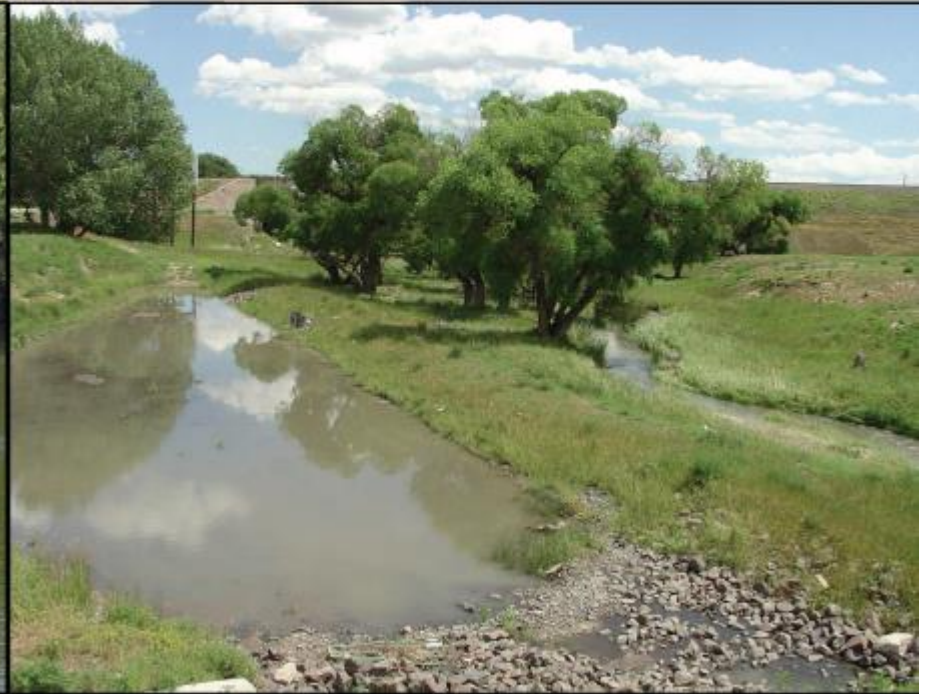
Detention ponds hold water for a short period of time; this pond temporarily holds water before it enters the stream.
